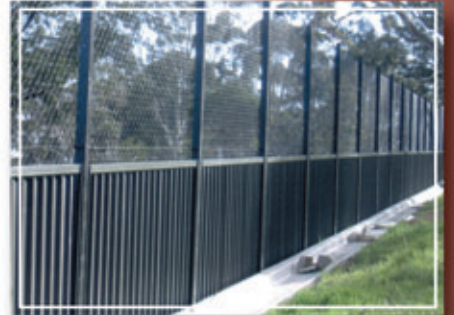
2400mm high combined Colorbond / chainmesh fence around wildlife reserve. Springthorpe Estate, Macleod
