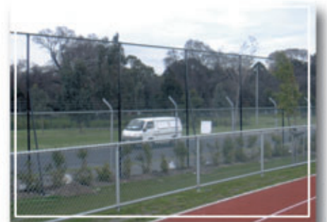
3600mm high black chainmesh safety fence.
