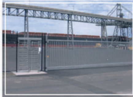
Security fencing and turnstiles. Port of Melbourne Corporation.
