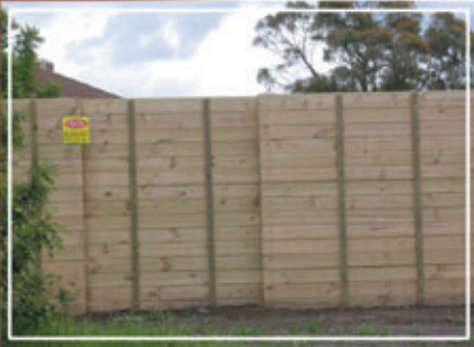
Sound attenuation fence. Hume Hwy, Craigieburn.
